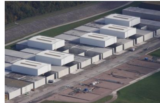
Example of a repository for surface disposal
