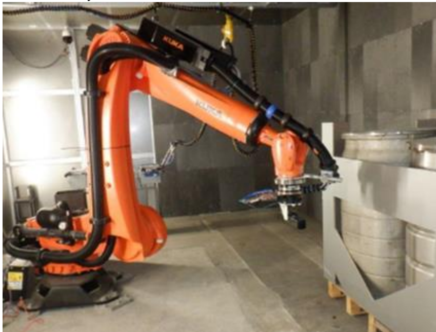
Fig. 8: A KUKA robot deploying a 3D Phoxi laser scanner to inspect a deformed ILW 500L Magnox drum while stored inside mock stillages at the NNL facility.
