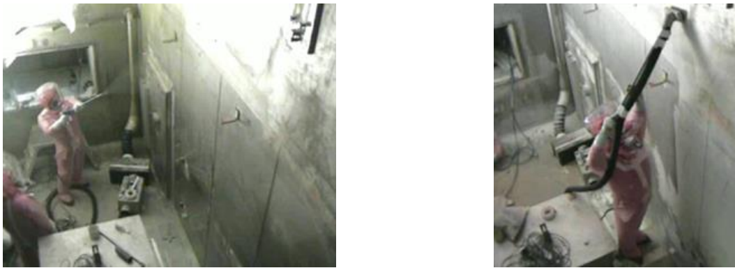
Figure 2. Spraying of a vacuumable gel on a SS surface (left) and vacuum cleaning of the solid waste after drying (right).
