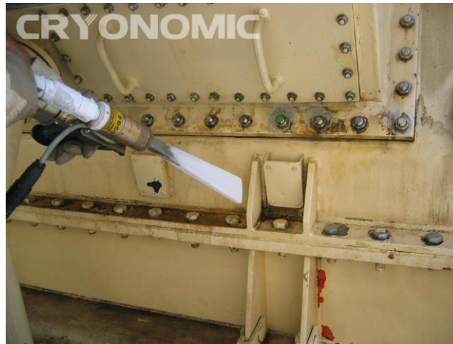
Figure 1: Nuclear decontamination with CRYONOMIC dry ice cleaning machine [2]
