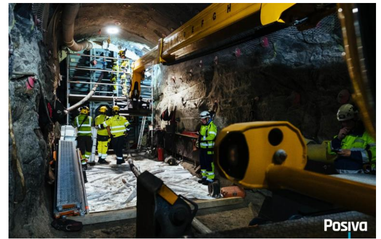
Finland - Trial Run of Final Disposal
