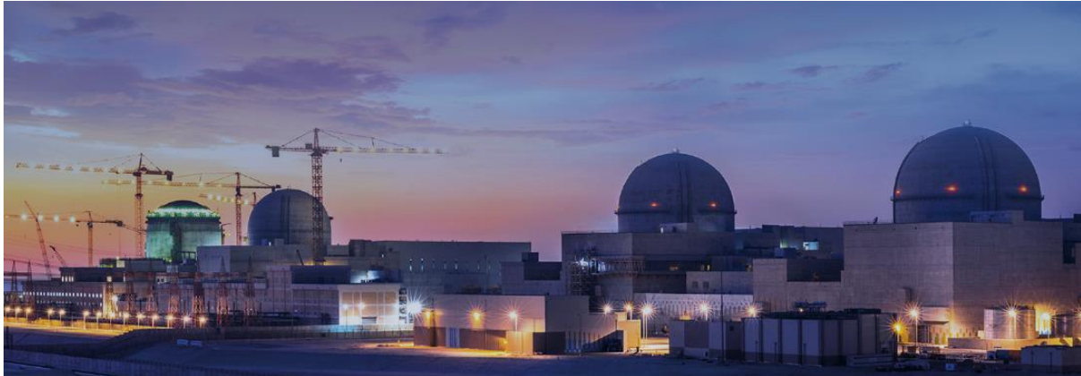
Figure 6.3 The four-unit Barakah nuclear power plant in the UAE. Image courtesy of Emirates Nuclear Energy Corporation
